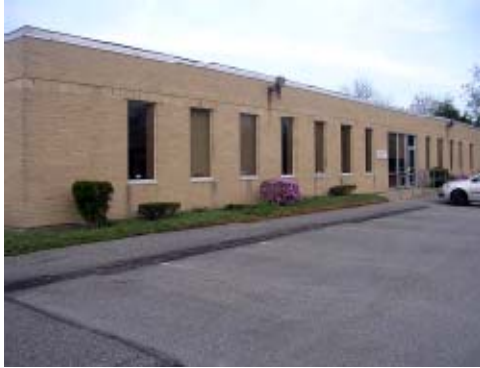
Exterior Wall 1 Entry Overview
