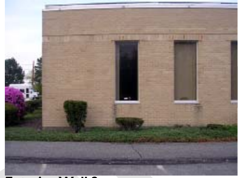
Exterior Wall 2 Wall at corner/end
