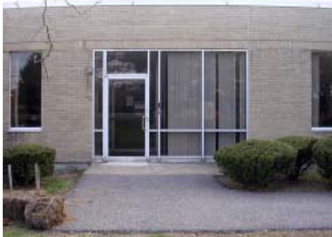
Exterior Wall 3 Main Entry Storefront
