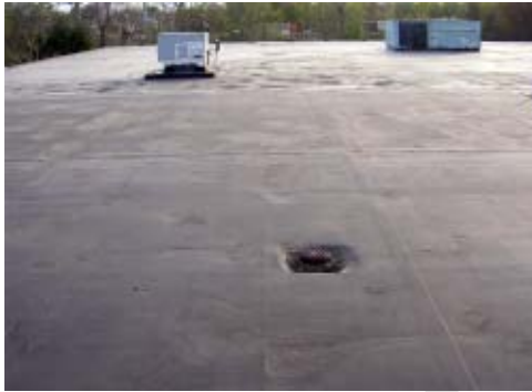
Roof 3 Typical Roof Drain
