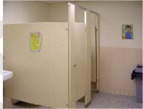
Toilet Rooms 2 Typical Stalls
