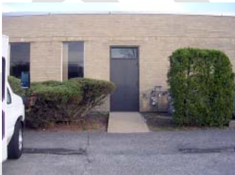
Exterior Wall 5 Secondary Exit Door
